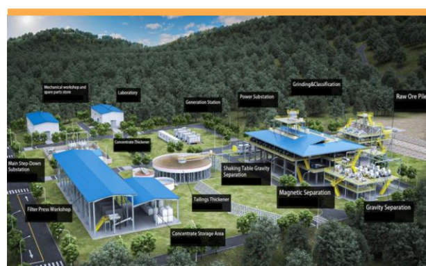
Kangankunde Processing Plant (Stage 1)
